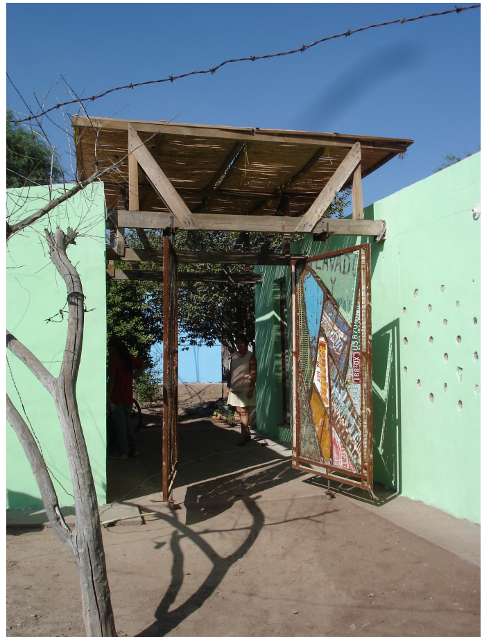
Figure 2: Entry utilizing re-used metal collected from local landfill, native carrizo shade structure and earthen adobe walls. Mexico.
